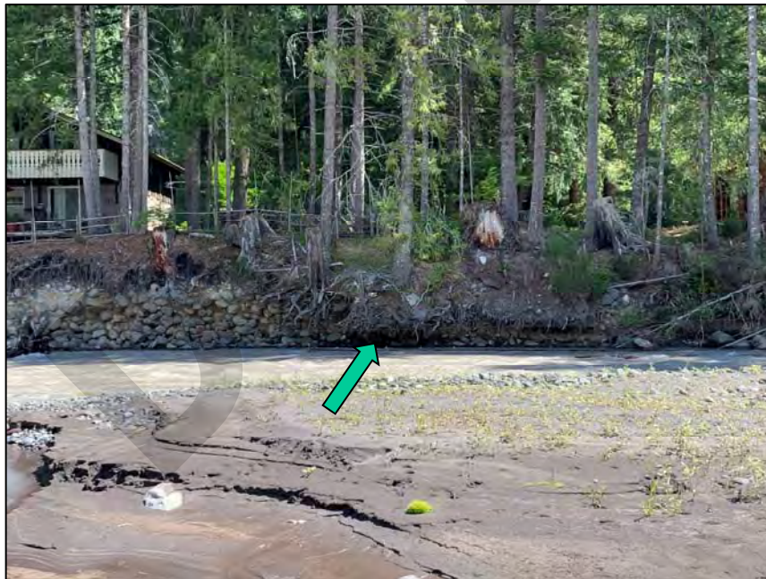
Photograph 18. Debris flow of unknown origin and significantly undercut bank. Tree growing atop of undercut with overhanging roots and other vegetation.
