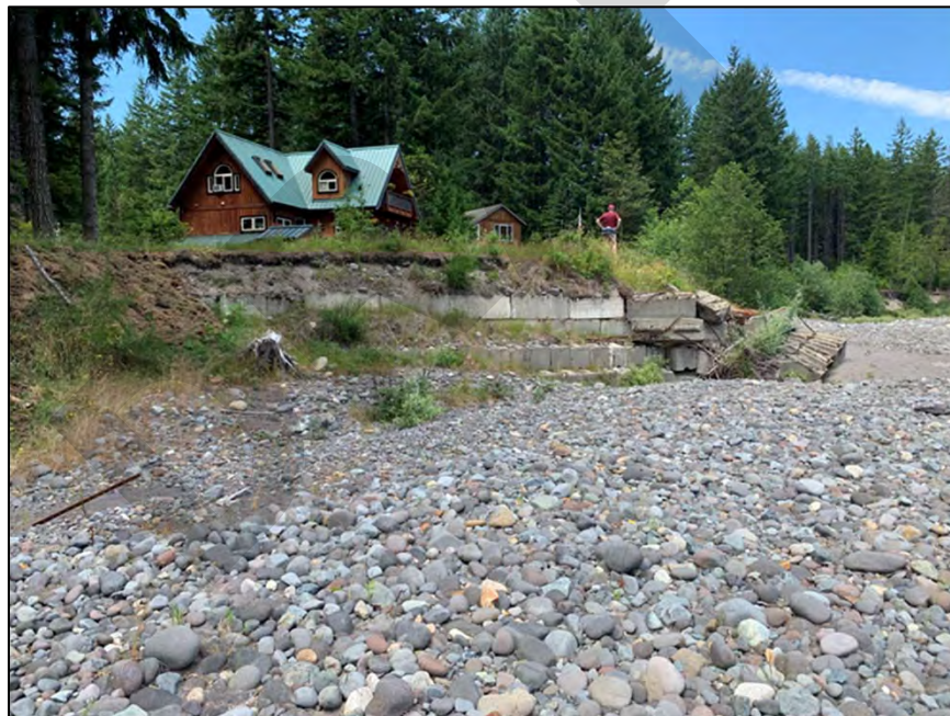
Photograph 14. Large ecology block revetment near RM 49.8.
