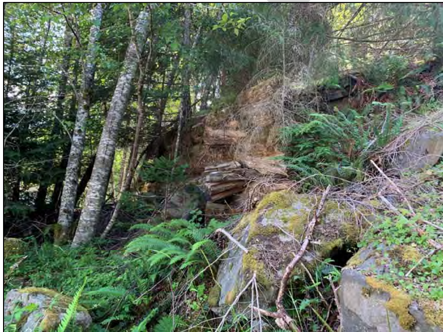
Photograph 10. Abutment to old bridge near RM 49.7 consists of massive riprap and wood.
