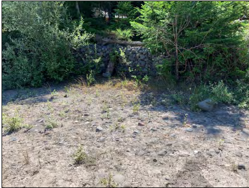
Photograph 15. Gabion basket revetment near RM 49.5.
